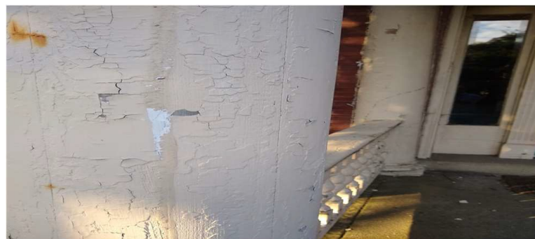
Photo 9: Porch components with deteriorated LBP.
