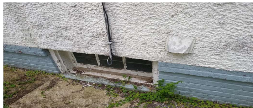
Photo 10: Foundation window with deteriorated LBP.
