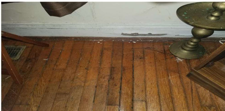
Photo 7: Baseboard with deteriorated lead-based paint (LBP).
