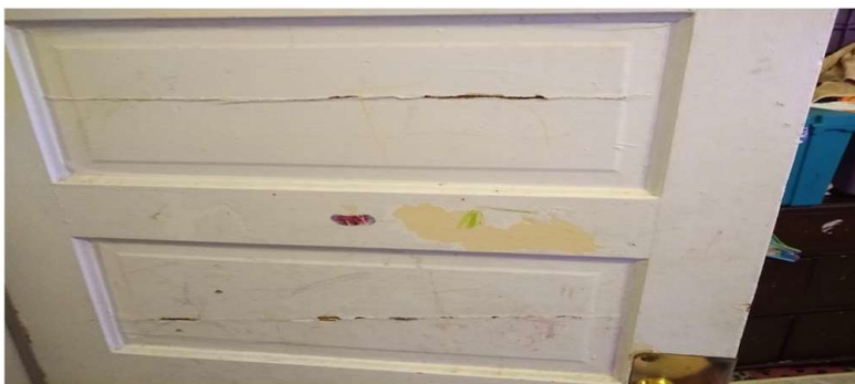
Photo 5: Door with deteriorated LBP.
