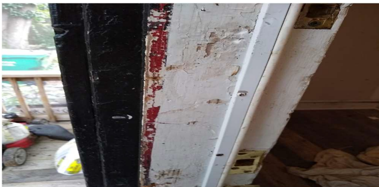
Photo 3: Typical front door jamb with deteriorated lead-based paint (LBP).
