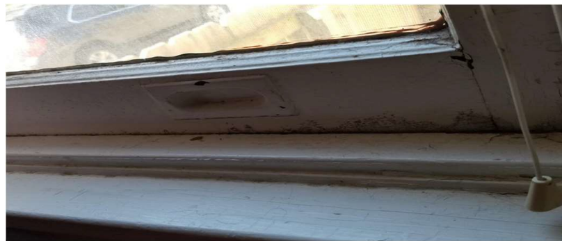
Photo 6: Deteriorated window and sill with deteriorated LBP.
