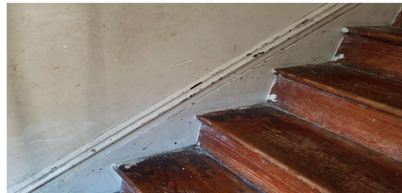
Photo 8: Stairway stringer with deteriorated LBP.
